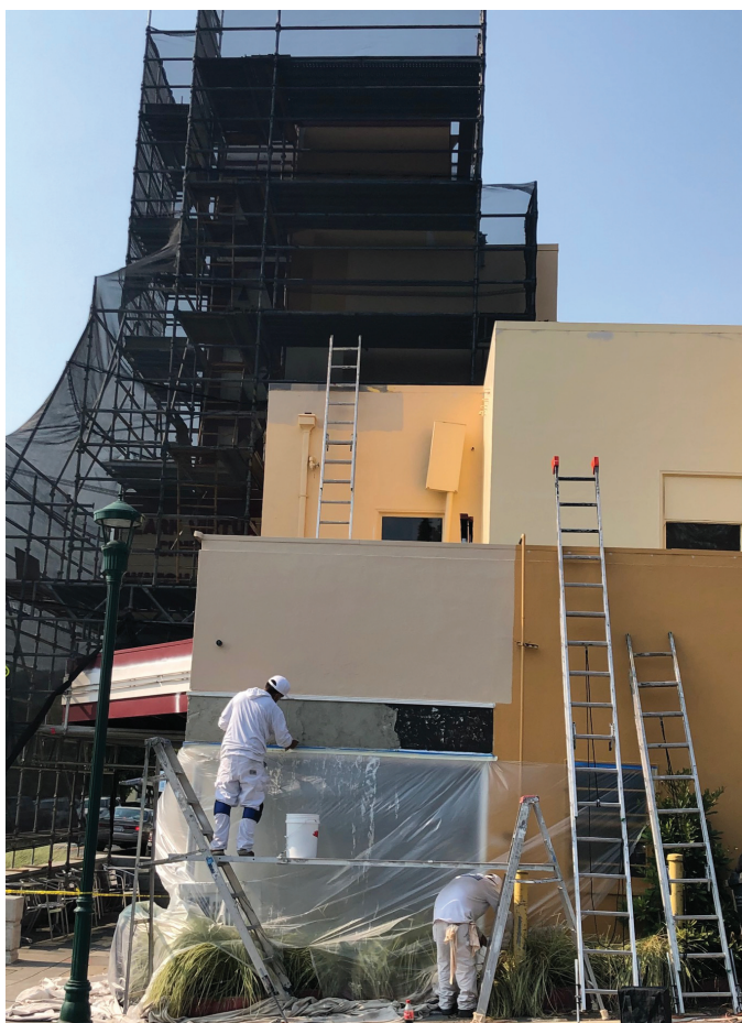
Working on the building exterior.
