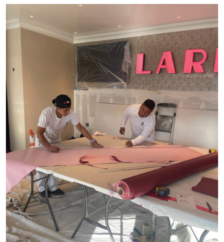
Measuring and cutting for the wallcovering installation.
