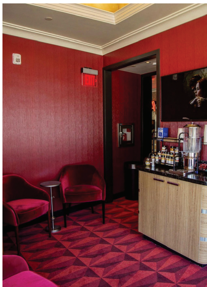
The deep red wallcovering was installed over a matching tinted primer.
